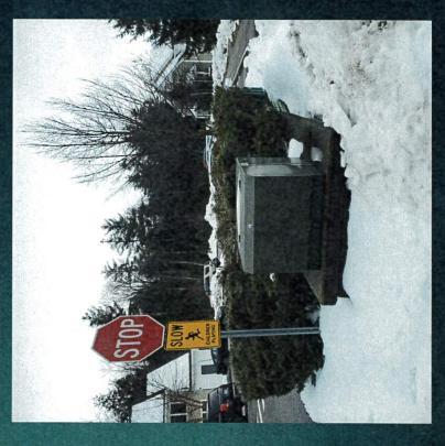
Two (2) Primary Sectionalizing/Junction Cabinets on 4'x 8' subsurface Concrete Vaults.
