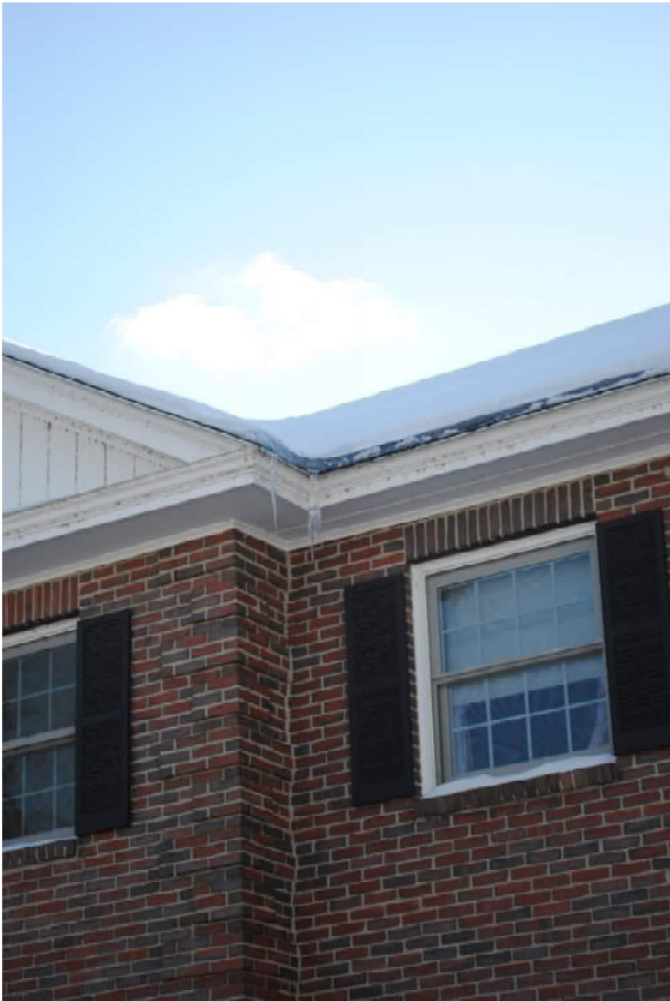
Minor ice damming at East façade roof
