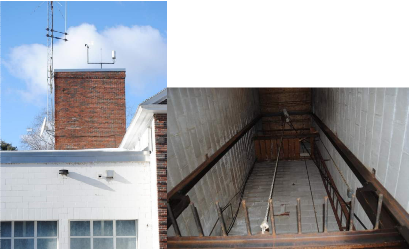
Hose tower exterior and interior views of moisture saturation.
