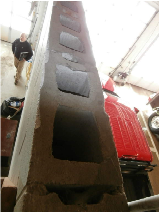
Top: Sally port interior wall, ungrouted and unreinforced / Bottom: South side entry canopy
