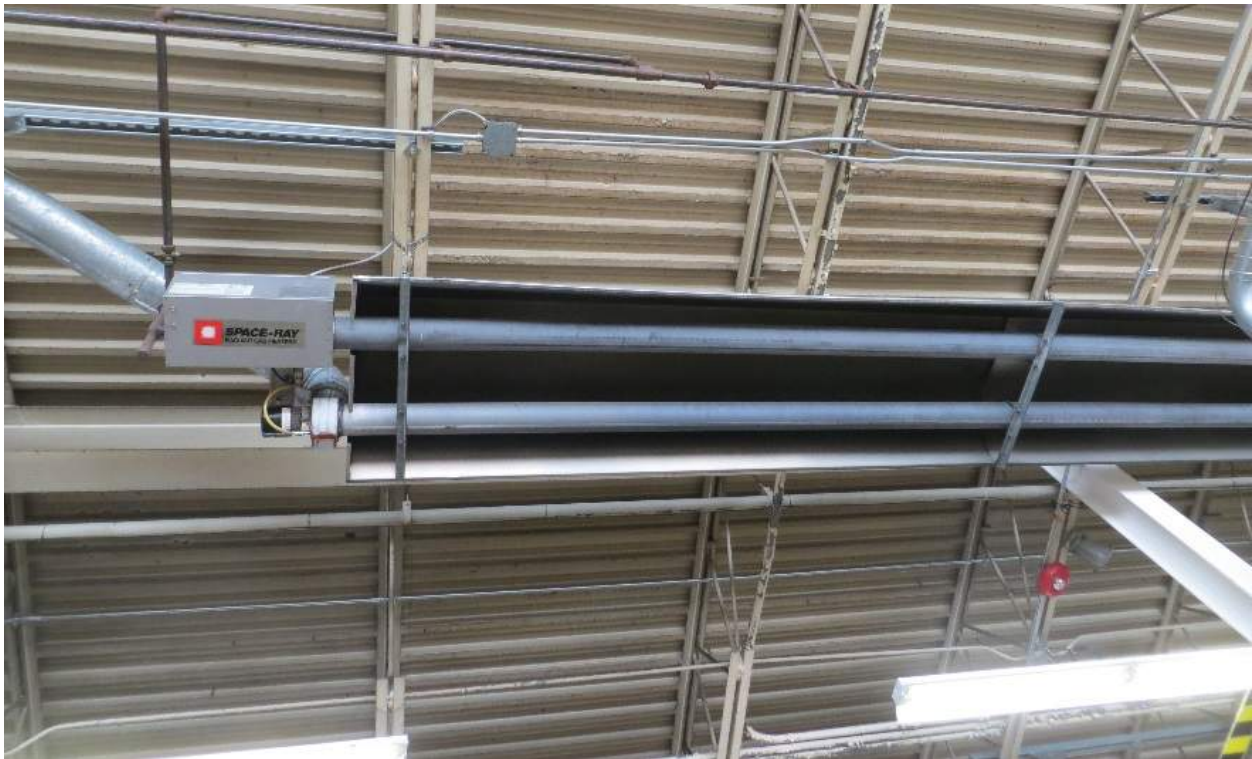
Example of Infrared Tube Heaters
