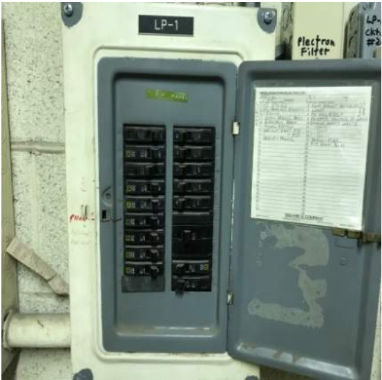
Circuit Breaker Panelboards
