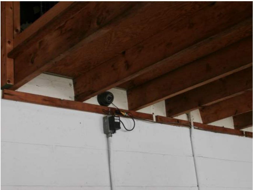
Sally port mezzanine framing ledger.
