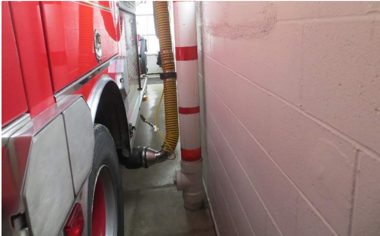
Vehicle Exhaust System Connected to Fire Truck
