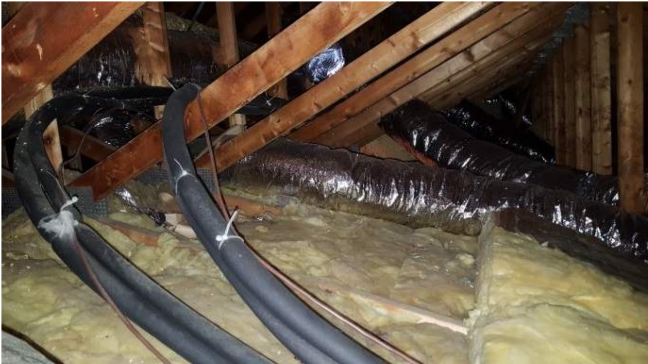
Existing Ductwork in Attic
