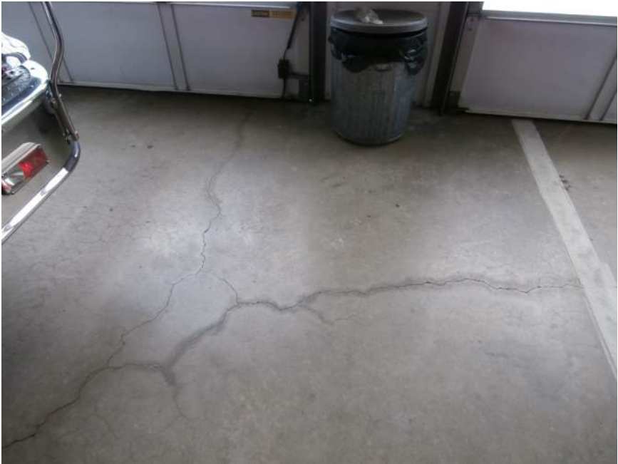
Cracked floor slab, Apparatus Bay
