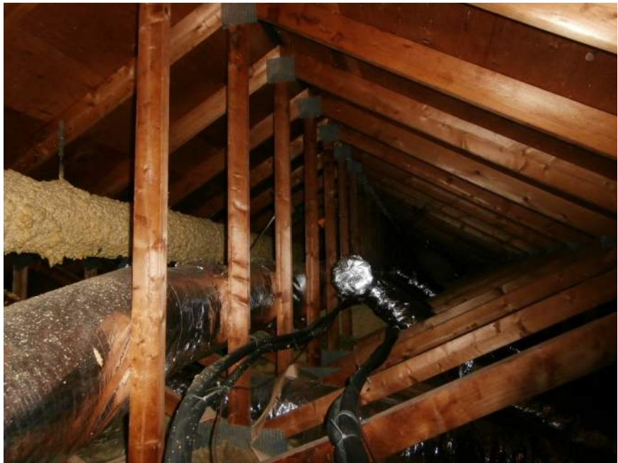
Scissor trusses – no thru-truss bracing
