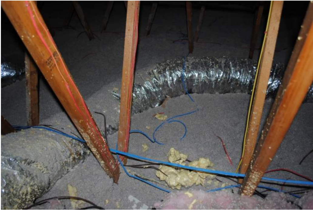
Loose blown-in cellulose insulation - uneven layered.
