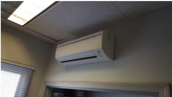
Ductless Split Serving Dispatch Room
