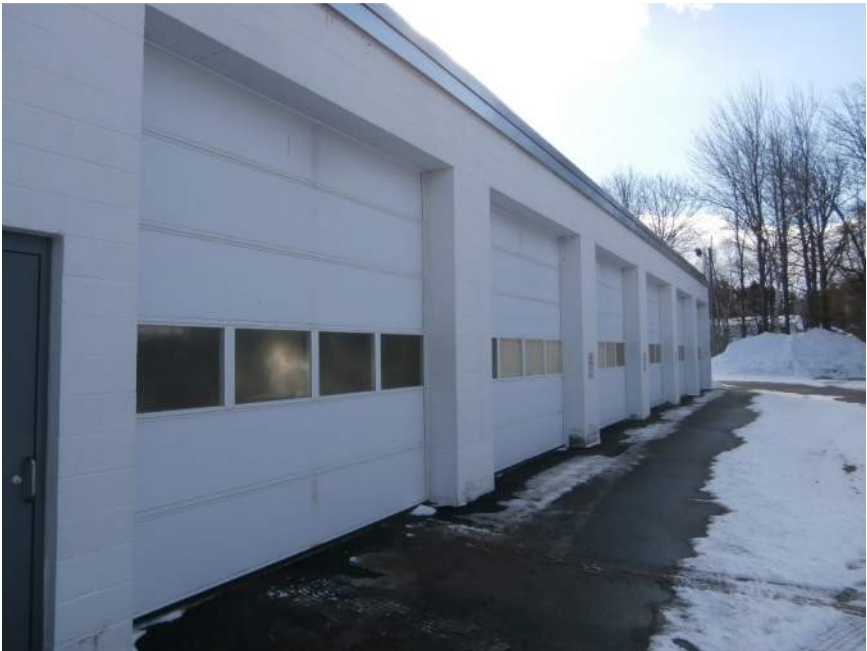
Reconstructed/Repaired masonry bearing walls and door headers, Apparatus Bay
