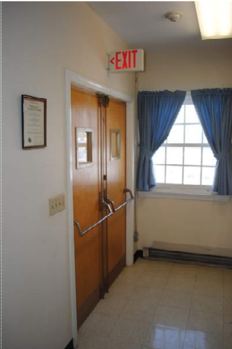
Missing door closer hardware
