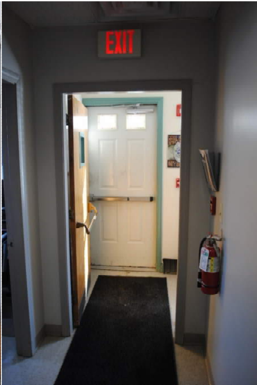
Door opening missing interior closers
