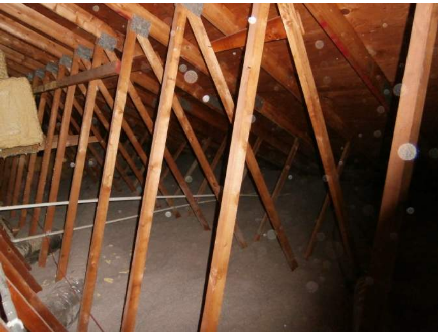
Fink roof truss 2x3 web members, no thru-truss bracing.
