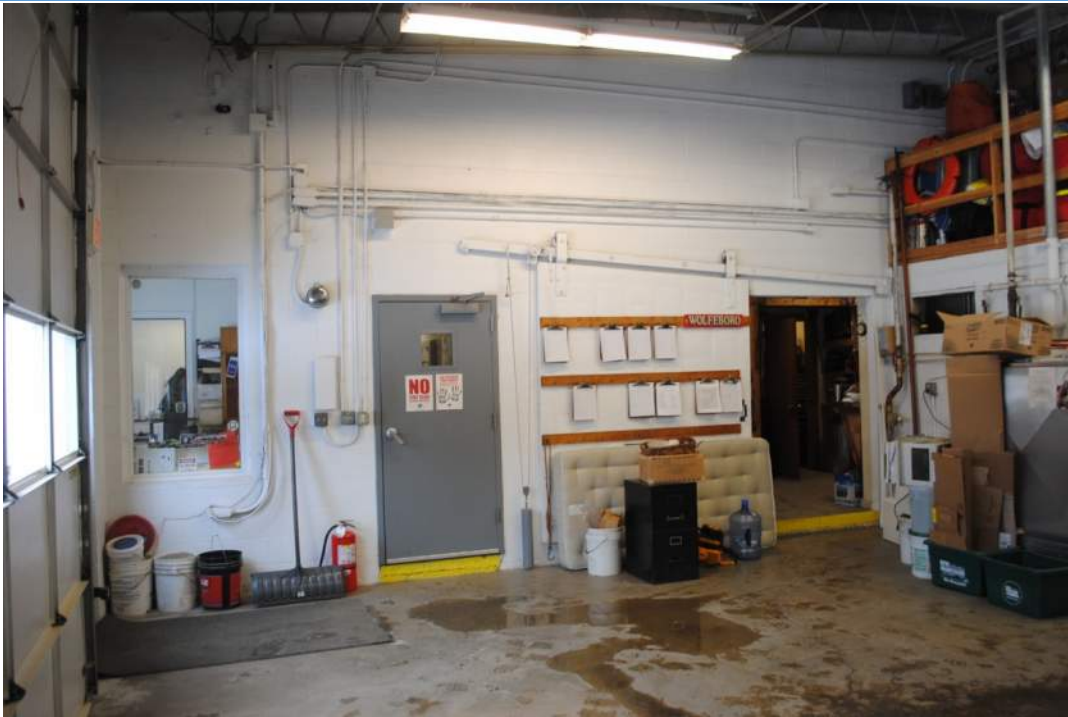
Fire Department Apparatus Bay (Storage Use Occupancy) block wall and rated sliding fire door. NOTE: window on left of wall is an unprotected opening through the concrete block separation wall into the Office (Business Use Occupancy)
