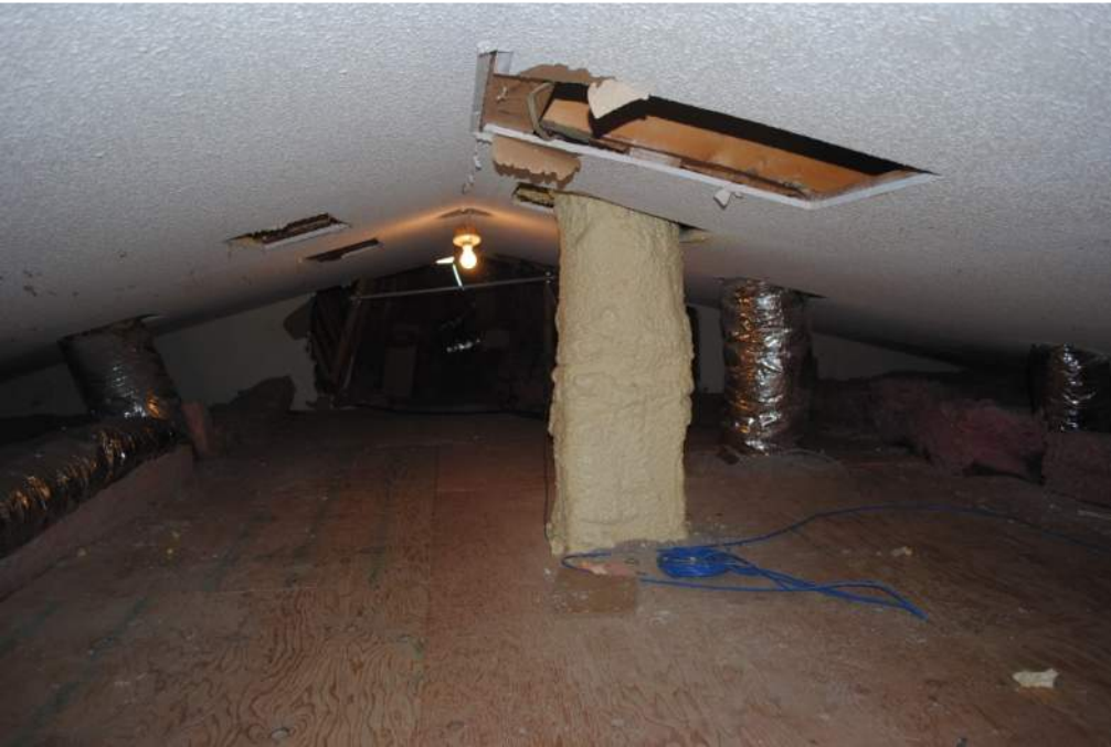
Scissor Truss area with plywood decking atop ceiling joists and openings to access H&V equipment controls.
