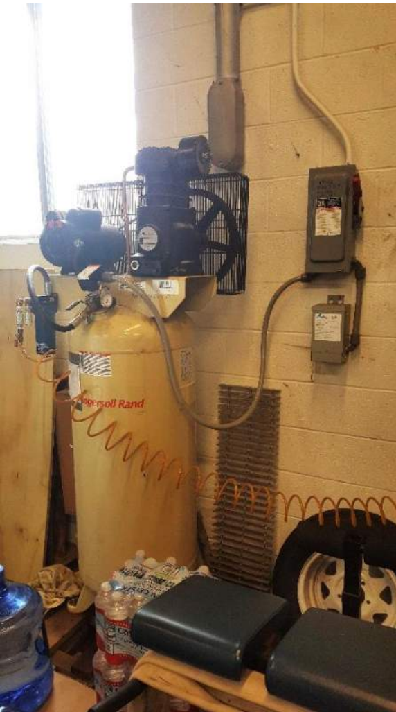
Existing Compressor Serving Plymovent Systems
