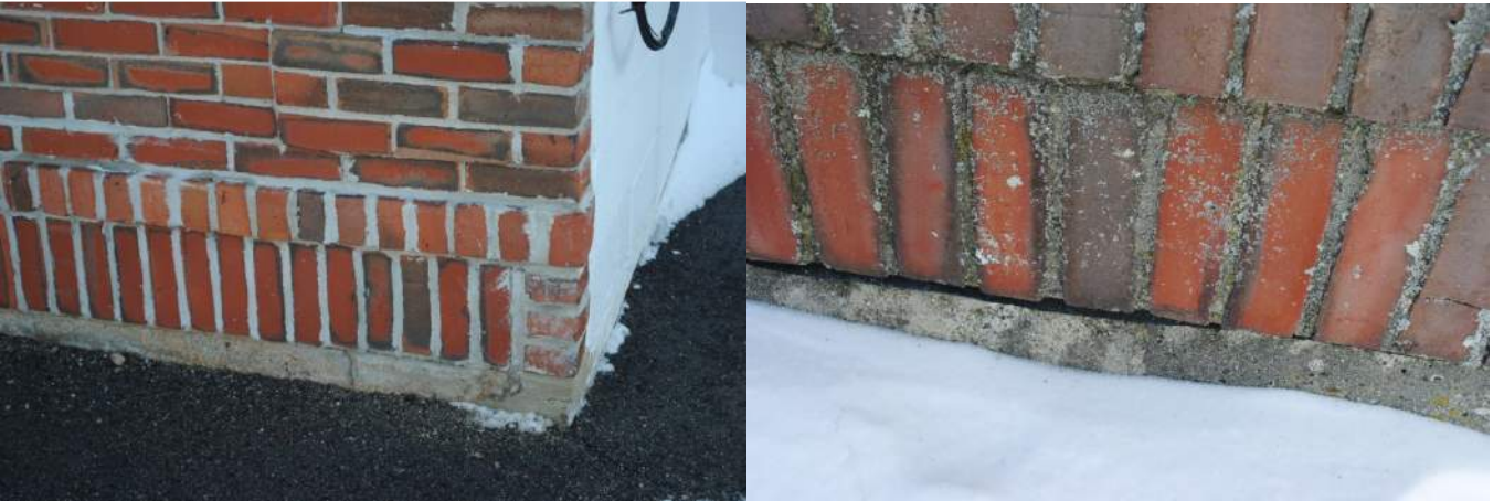
Brick masonry previous repointing – no brick weeps
