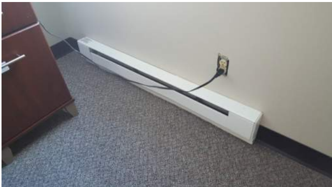
Example of Recently Installed Electric Baseboard
