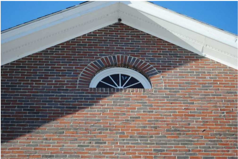
Missing sealant around window to brick joint.
