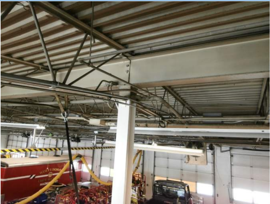
Open web joists and centerline steel framing, Apparatus Bay.
