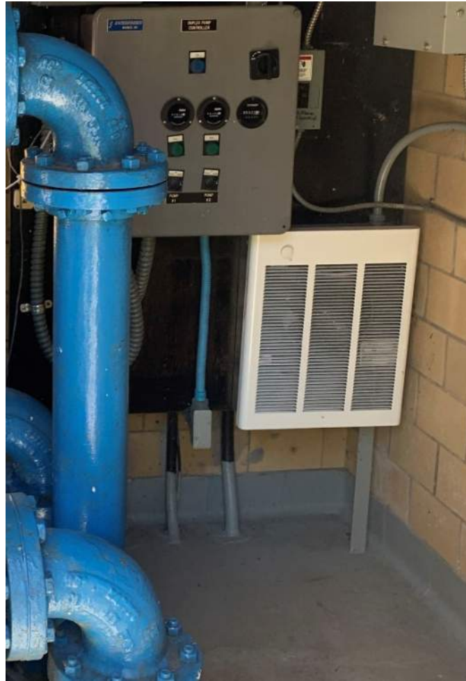
Figure 3-8 Lehner Street Pump Building Unit Heater
