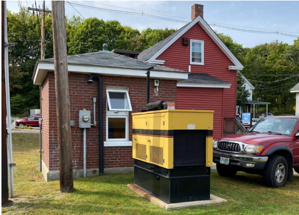
Figure 3-1 Lehner St. Pump Station with Emergency Generator
