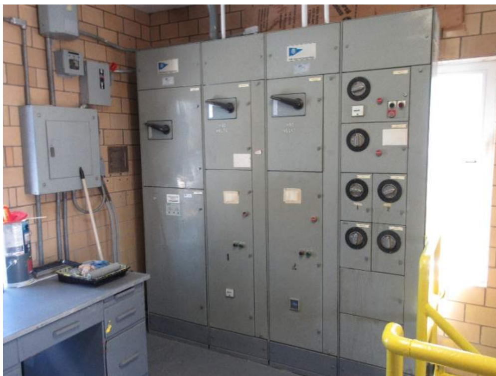
Figure 4-9 Motor Control Center (MCC)
