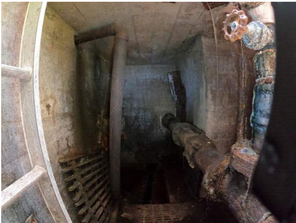
Figure 3-7 Corrosion in Main Wet Well
