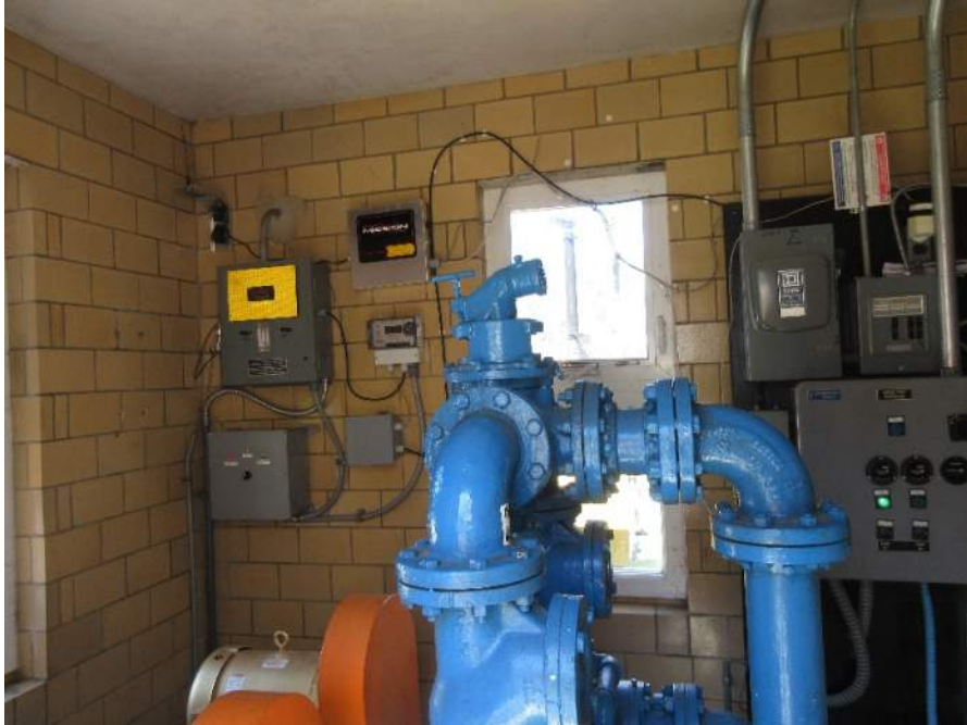
Figure 3-10 Pump Controller and Pump Control Panel
