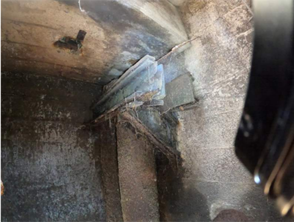
Figure 3-6 Exposed Reinforcement in Main Wet Well
