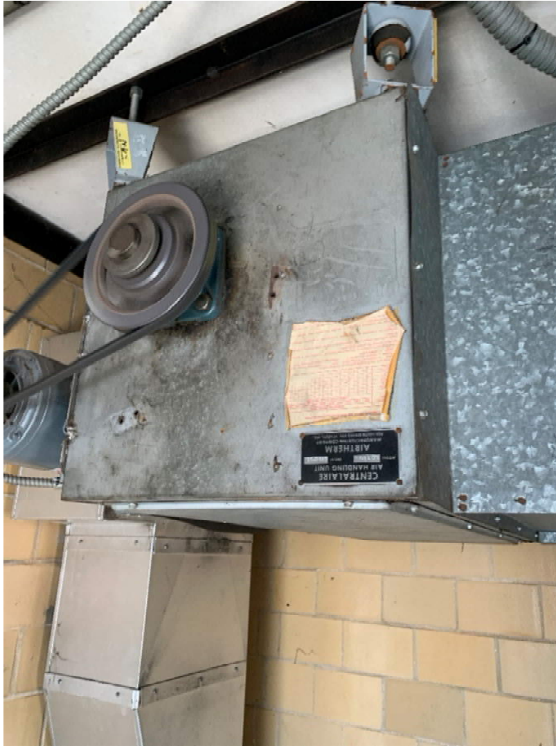
Figure 4-7 Ceiling Mounted Supply Fan with Inline Duct Heater
