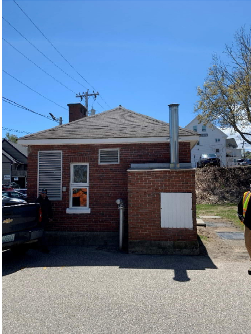
Figure 4-6 Exterior Louvers and Wet Well Ventilation Chase
