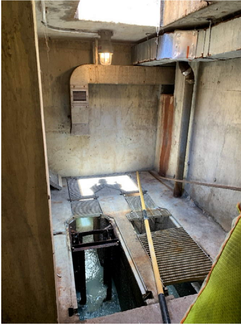
Figure 4-8 Wet Well Exhaust Ductwork
