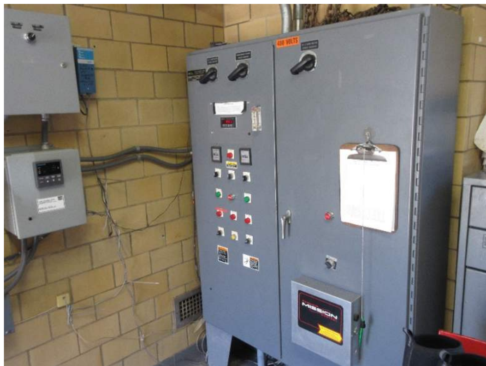
Figure 4-10 Pump Control Panel
