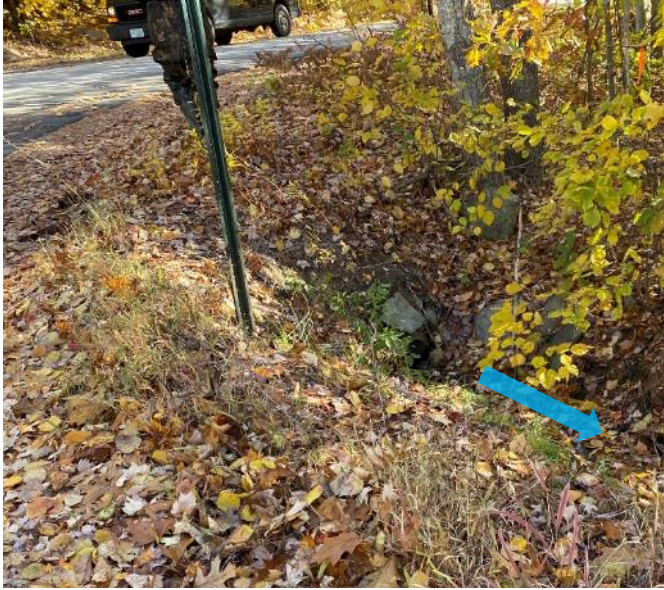
Photo 9: Culvert outlet at north end of Cross Road
