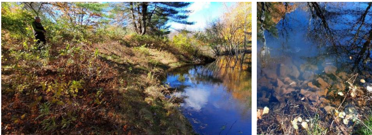
Photos 22 and 23: The bank stabilization area had a stabilized/ vegetated slope with stone armoring at the toe of slope.
