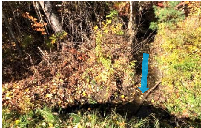
Photo 3: Culvert Inlet (view from road at Brewster Heights)
