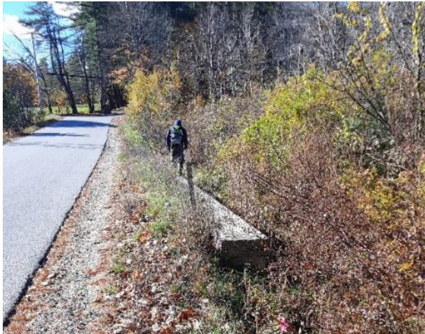
Photo 11: Upstream side of bridge/ culvert
