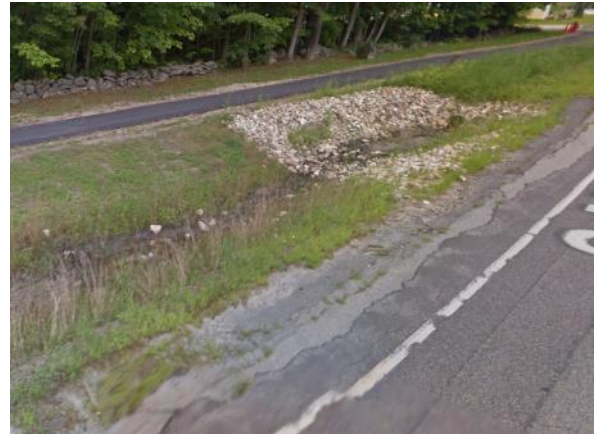
Photo 17: Drainage channel parallel to S Main St.
