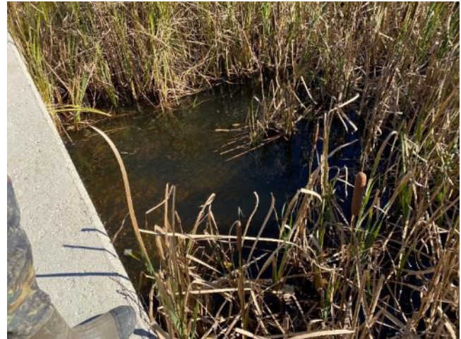
Photo 12: Downstream side of bridge culvert
