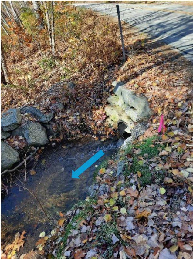
Photo 7: Culvert under Pleasant Valley Road
