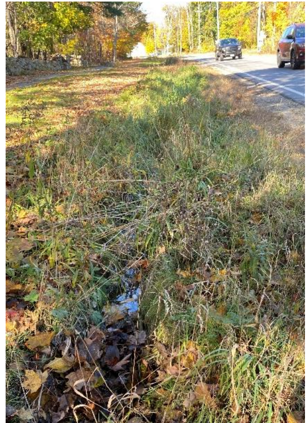
Photo 18: Drop catch basin location (buried)
