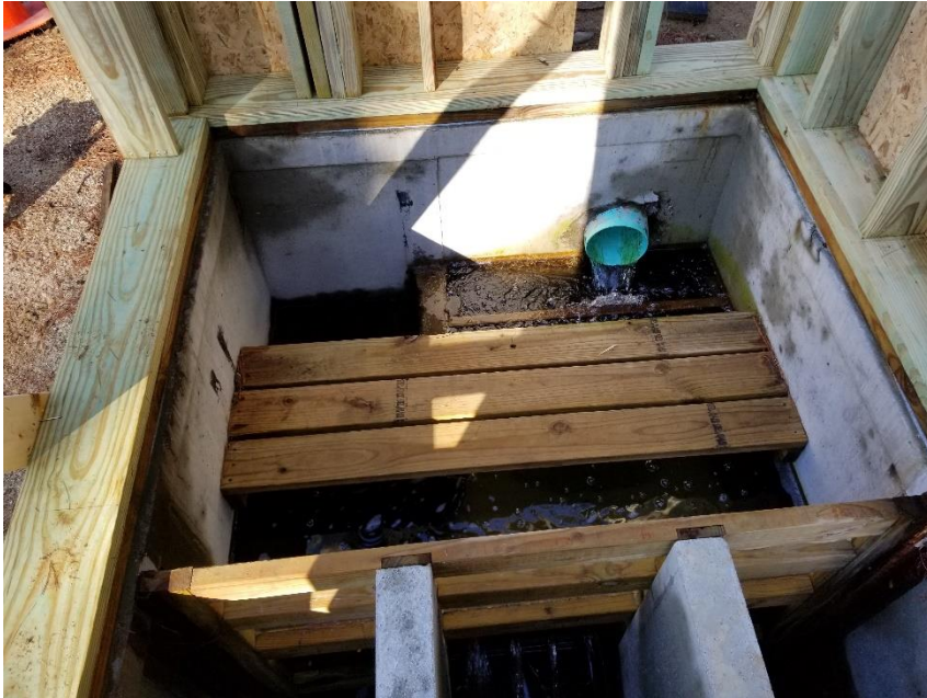
11: Looking into the central flow control structure (photo taken 11/25/19)
