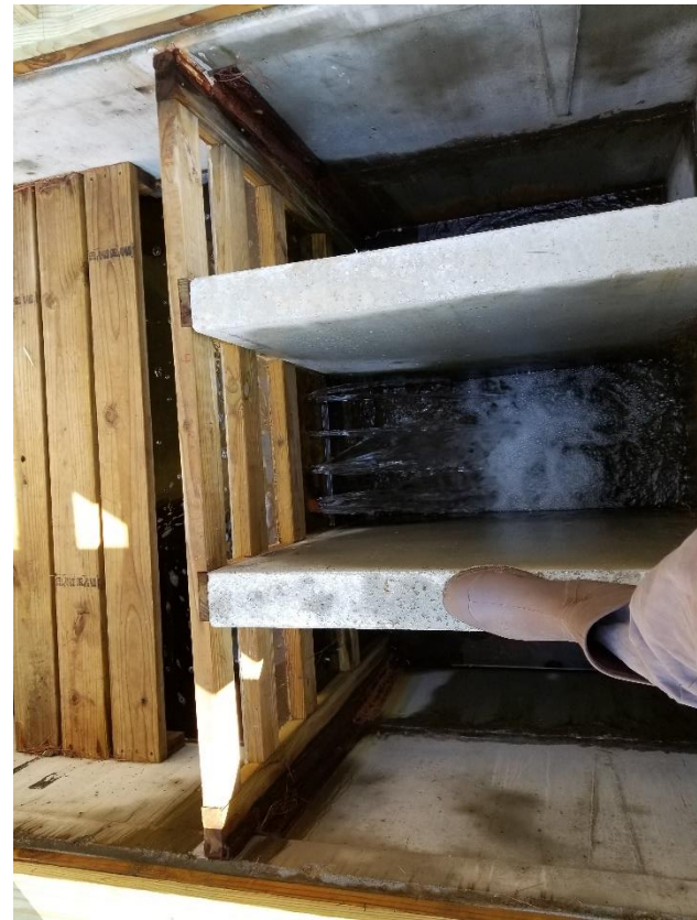
12: Looking into the central flow control structure (12/26/19)
