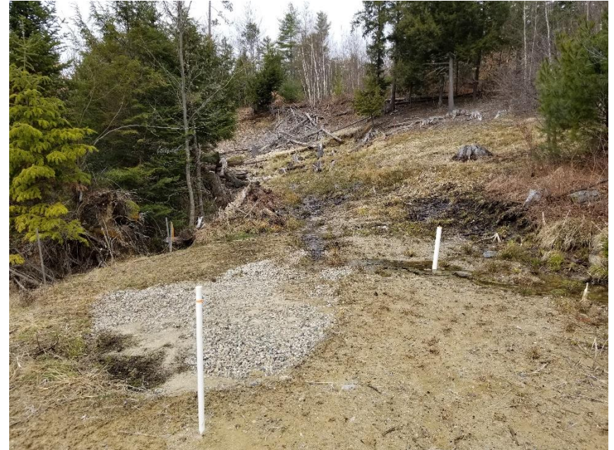
6: Looking northwest at the Central Seep area (4/2/20)
