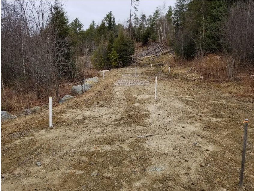
5: Looking northwest towards Cut-off Trench #2 (photo taken 4/2/20)
