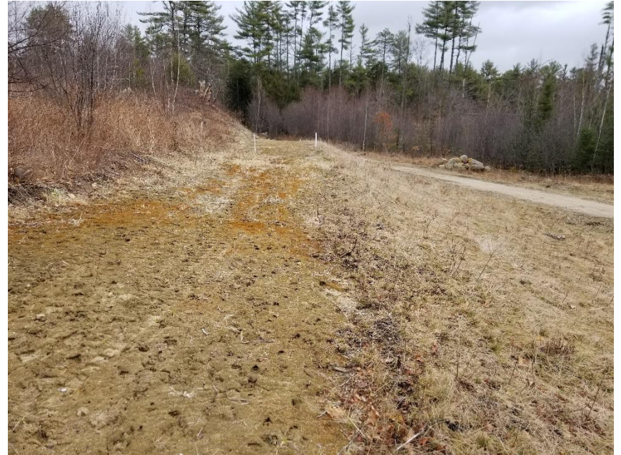
8: Looking east towards Cut-off Trench #1 (4/2/20)
