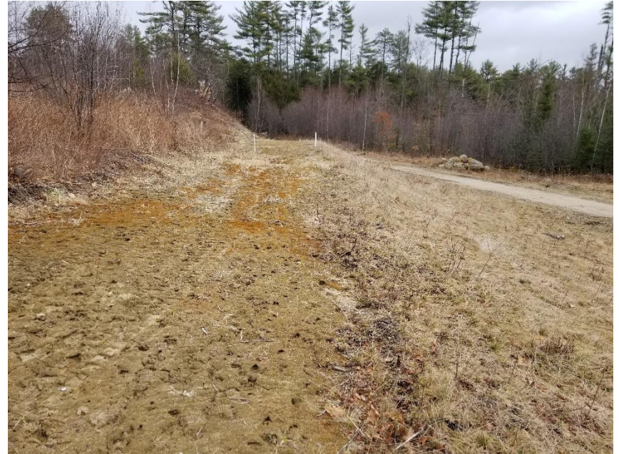
8: Looking east towards Cut-off Trench #1 (4/2/20)
