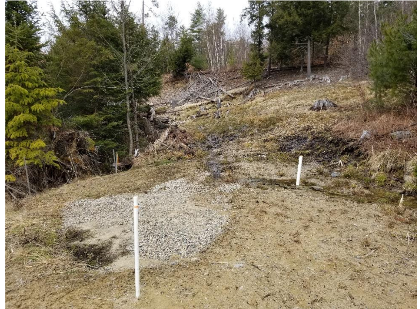
6: Looking northwest at the Central Seep area (4/2/20)
