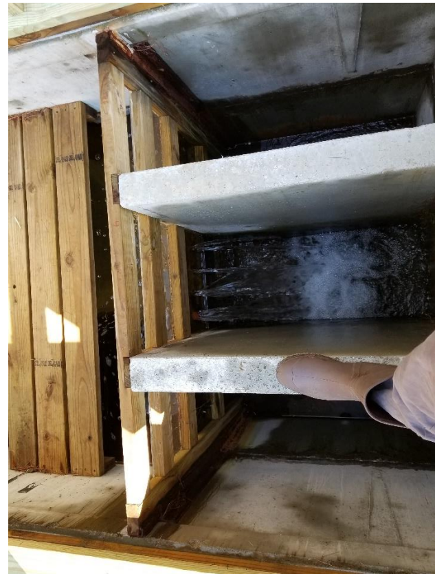
12: Looking into the central flow control structure (12/26/19)
