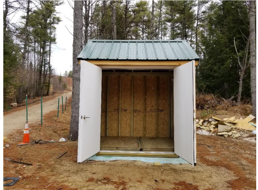
10: Looking east at the central flow control structure (4/2/20)
