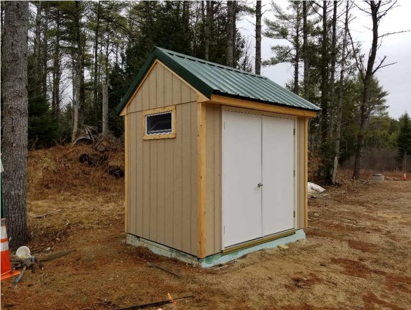
9: Looking east at the central flow control structure (photo taken 4/2/20)
