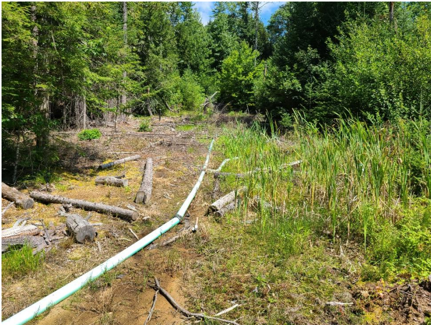
13: Looking northeast at the Western Seep area (photo taken 5/8/20)
