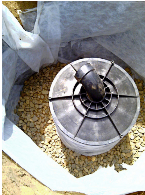
A commercially manufactured drywell being installed to capture water from roof downspout.
