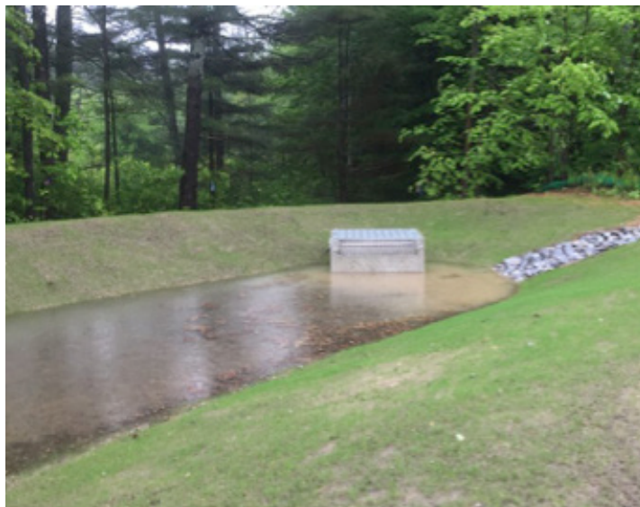
Stormwater retention and filtration system installed in the Crescent Lake watershed: shown before and immediately after a heavy rain.
