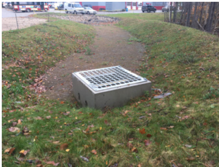
Stormwater retention and filtration system installed in the Crescent Lake watershed: shown before and immediately after a heavy rain.
