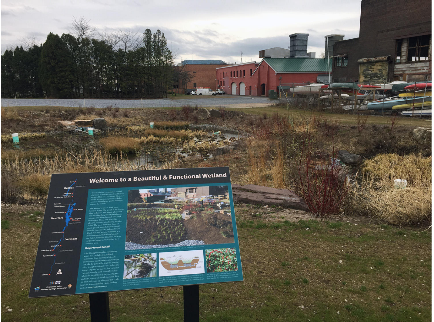
A subsurface gravel wetland system near the Andy Williams Skate Park on Burlington's waterfront captures and filters stormwater before it flows into Lake Champlain. Photo Credit Angela Evancie / VPR
