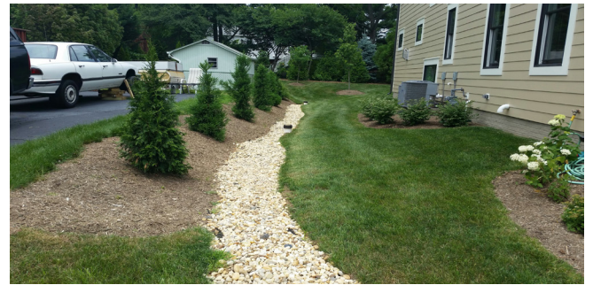
An infiltration trench intercepts and temporarily stores stormwater runoff and promotes infiltration. Photo credit: arlingtonva.us
