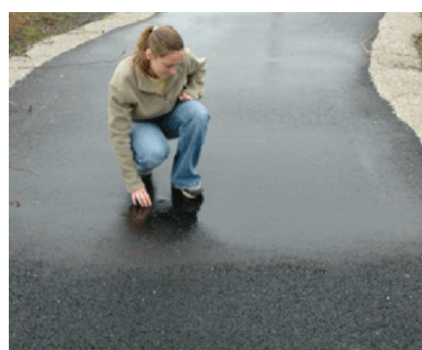
The line between porous and non-porous asphalt.
