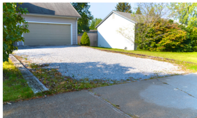
A gravel driveway with clean gravel and no wash-out
