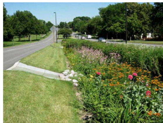
A roadside bioswale collects runoff from road.
