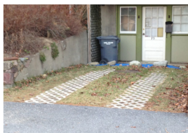
A concrete paver ribbon driveway.
