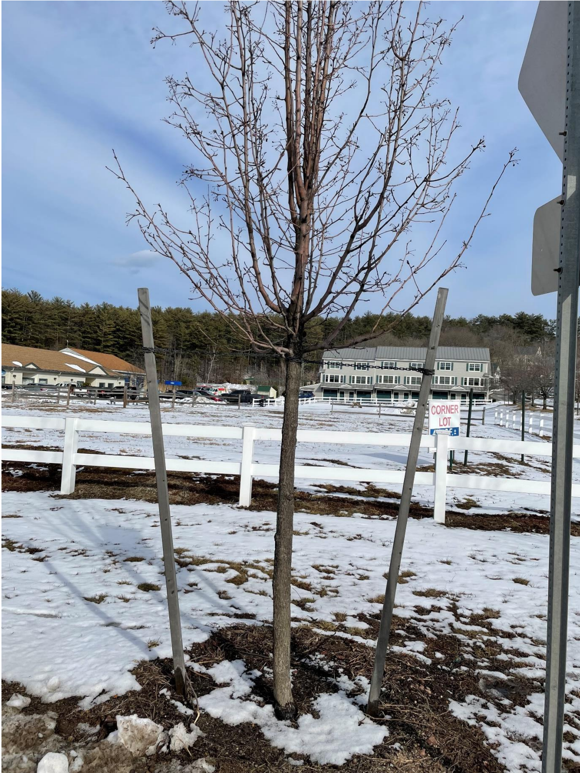
Tree #80 recommended for inspection and potential removal of tree guy/staking system. Staking newly planted trees for too long is a common issue in young trees. Trees should not be staked past approximately six months following planting.
