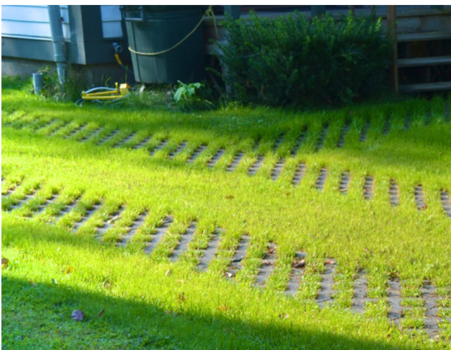
Stormwater friendly driveways like this one, where an open concrete paver system was planted with grass, offer multiple benefits for homeowners, local infrastructure, and nearby lake water quality.
