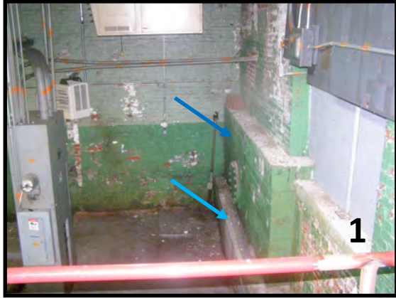
1. Photo of the original building foundation wall and footing, from the north end; 2. Various floor materials in the south end; 3, 4 & 5. View inside various pits; 6. Raised sections of floor at north end of building.
