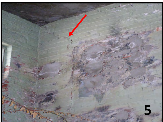
1. Dividing wall between north and south ends (original exterior north-wall of 1897 building), viewed from the south; 2. Close up of same wall adjacent to window—shows displacement and deterioration.; 3. East wall of south end of the building; 4. East wall at the north end of the building; 5. Close up of east wall at south section (portion of 1897 structure), again there are signs of displacement and deterioration; 6. Close up of deterioration of the dividing wall viewed from the north end.
