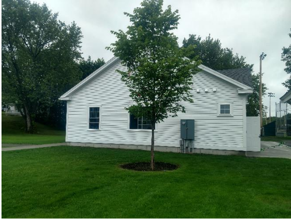
Foss Field Pavilion finished in time for the Summer Season 2018!
